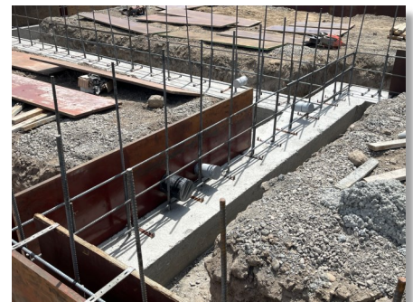
City of Toppenish Solids Handling Treatment Upgrade
