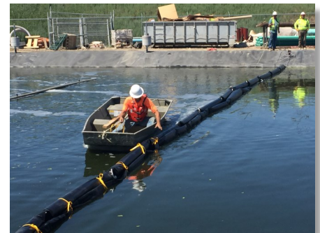
Town of Harrah Wastewater Treatment Plant Upgrades
